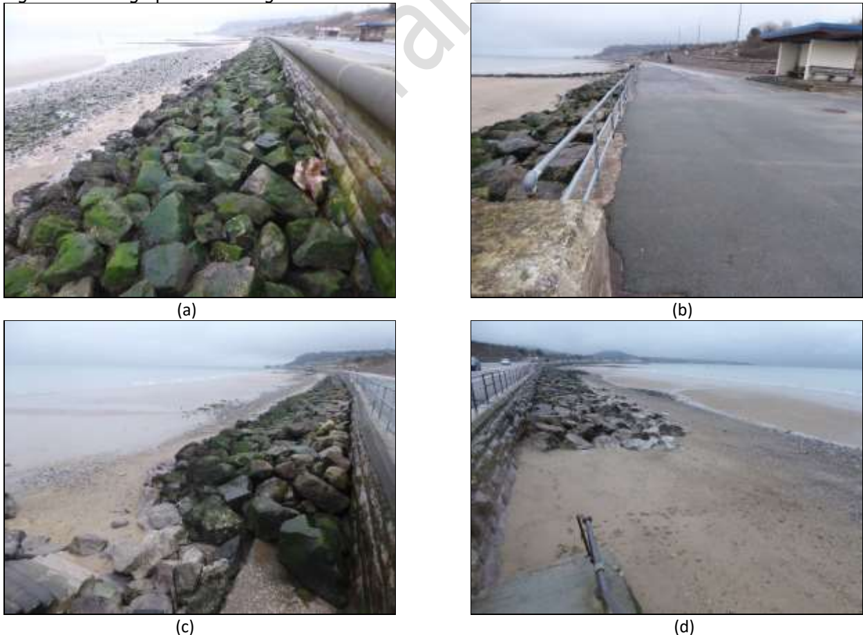
Figure 4: Photographs of Existing Coastal Defences and Promenade
