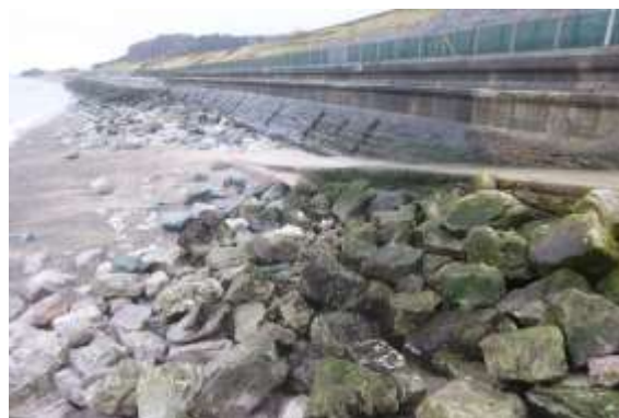
Foreshore Access at Beach Rd/Cliff Gardens
