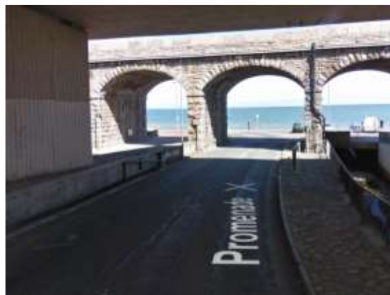
(R) Promenade/Cliff Gardens Junction
